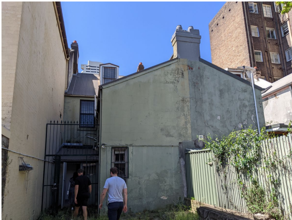
rear of terrace viewed from rear courtyard
