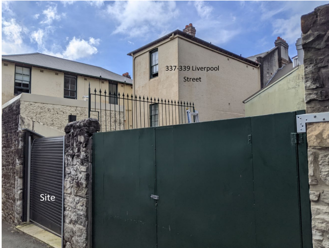
rear of site looking towards adjacent flat building at 337-339 Liverpool Street
