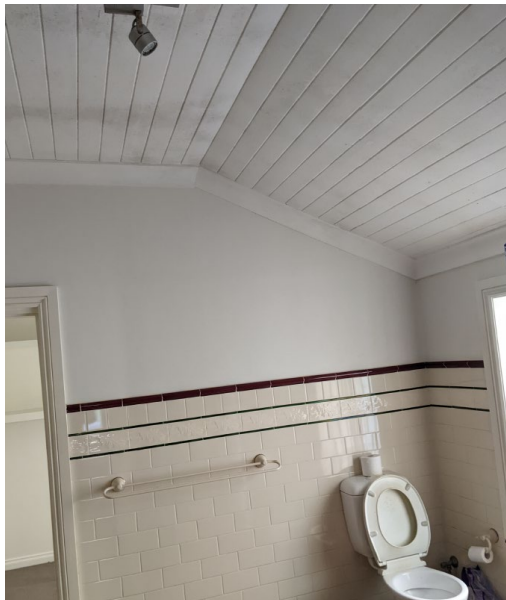
first floor rear wing
